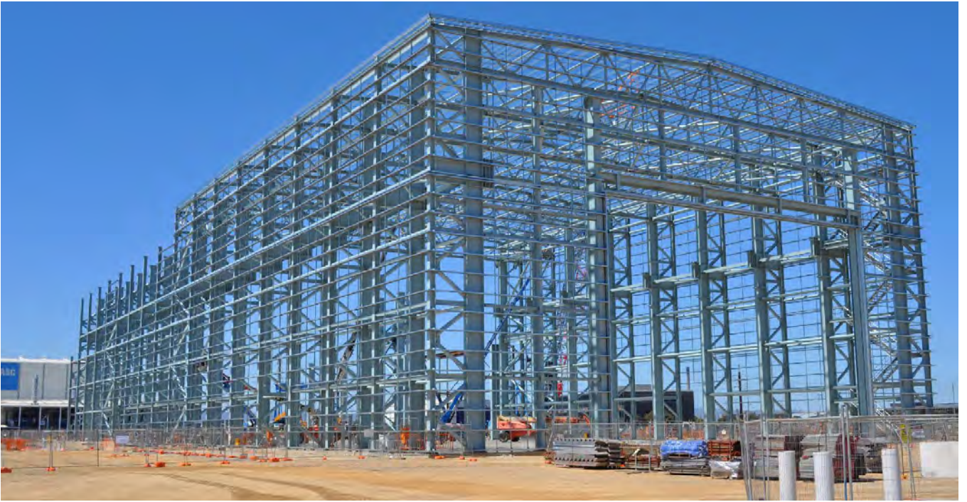
Photo 5 Photo showing steel skeleton / superstructure of a building at Osborne Naval Shipyard (Source: ANI supplied)
