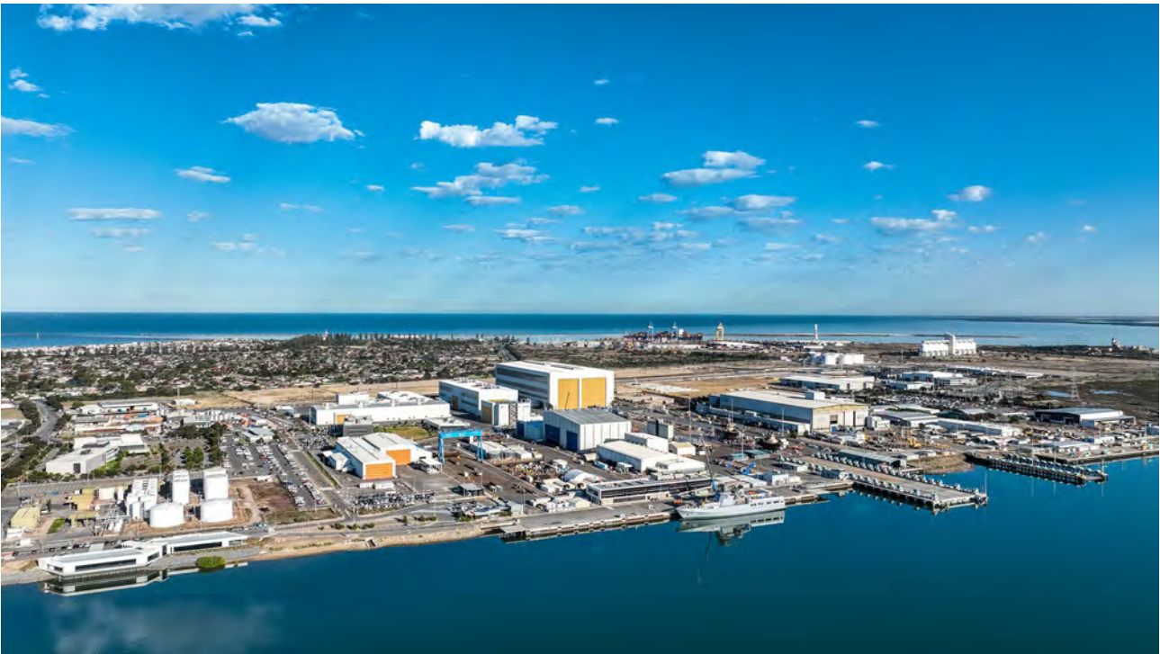
Figure 31 Visual example of structures to be built within the Submarine Construction Yard (Source: ANI 2023)
