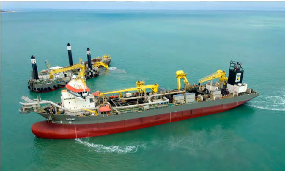
Photo 12 Trailing Suction Hopper Dredge Gateway and Backhoe Dredge Magnor in Gulf St Vincent (Source: Boskalis 2020)
